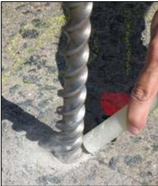
Figure 9: Drilled Powder Sampling on a Bridge Deck.
