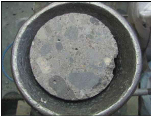
Figure 12: Pulverized Concrete Core
