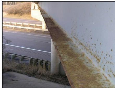
Element: Fascia Beams (View B) Condition State: 3 (Poor) >3 – 16% corrosion/defects
