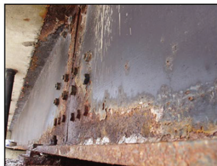
Element: Fascia Beams (View B) Condition State: 4 (Severe) >16% corrosion/defects
