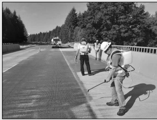
Spray Applied Waterproofing
