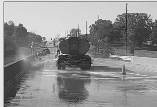
Watering the Bridge Deck and Jersey Barriers
