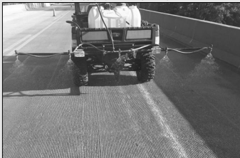
Spray Applying the Waterproofing
