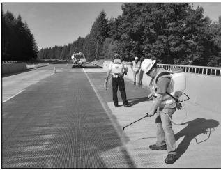
Spray Applied Waterproofing
