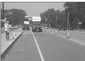
Drying after Application
