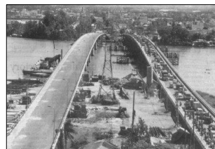
Binh Trieu Bridge – Ho Chi Minh City, Vietnam
