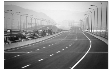
New Construction Freeway – Taipei, Taiwan 65,000 square meters
