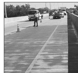
Spray Applied Waterproofing
