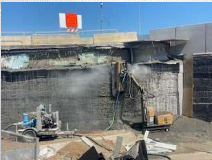
4" to 7" Fascia Removals
