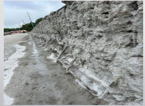
Hydrodemolished Wall
