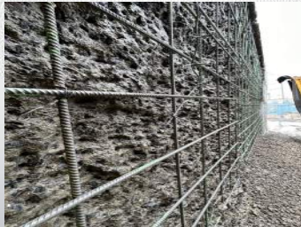
4" to 7" Fascia Removals
