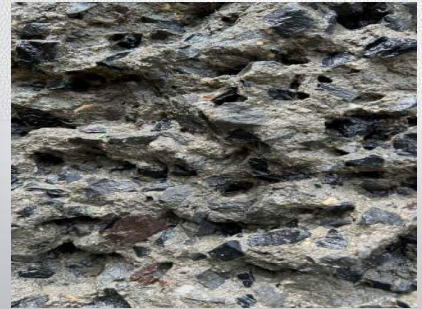
4" to 7" Fascia Removals
