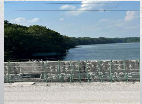
Dowel/Rebar Installation
