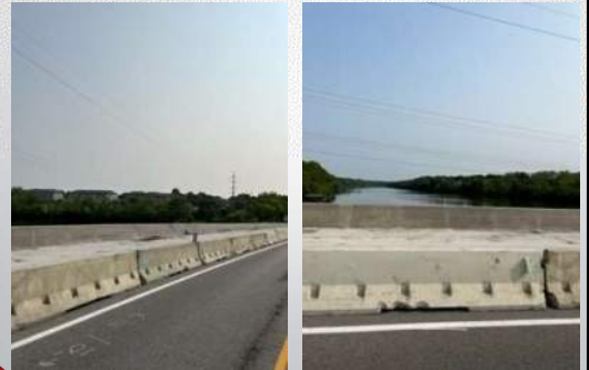
Refaced Parapet Wall
