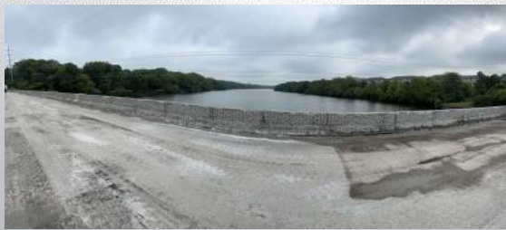
Hydrodemolished Wall
