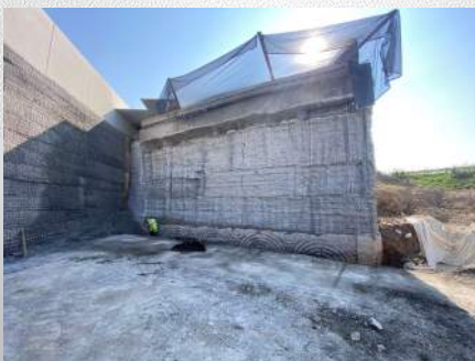
Almost Completed Abutment 3
