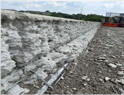
Hydrodemolished Wall
