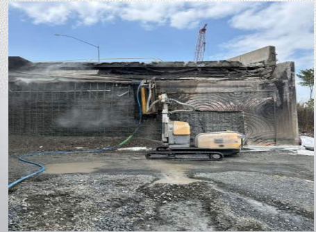
4" to 7" Fascia Removals
