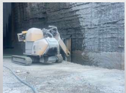
Additional Removals Abutment 3
