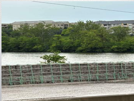
Dowel/Rebar Installation
