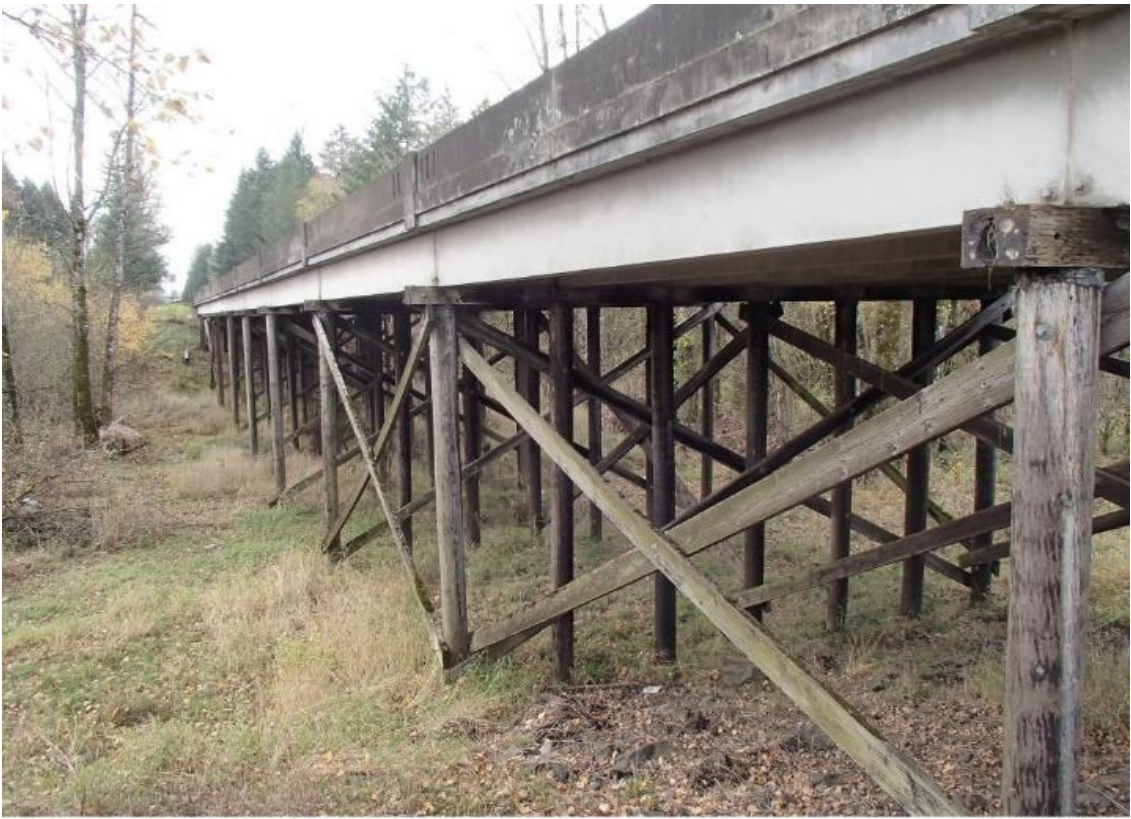
YAMHILL RIVER OVERFLOW - BR# 08492 - HWY 39 - MP: 45.76
