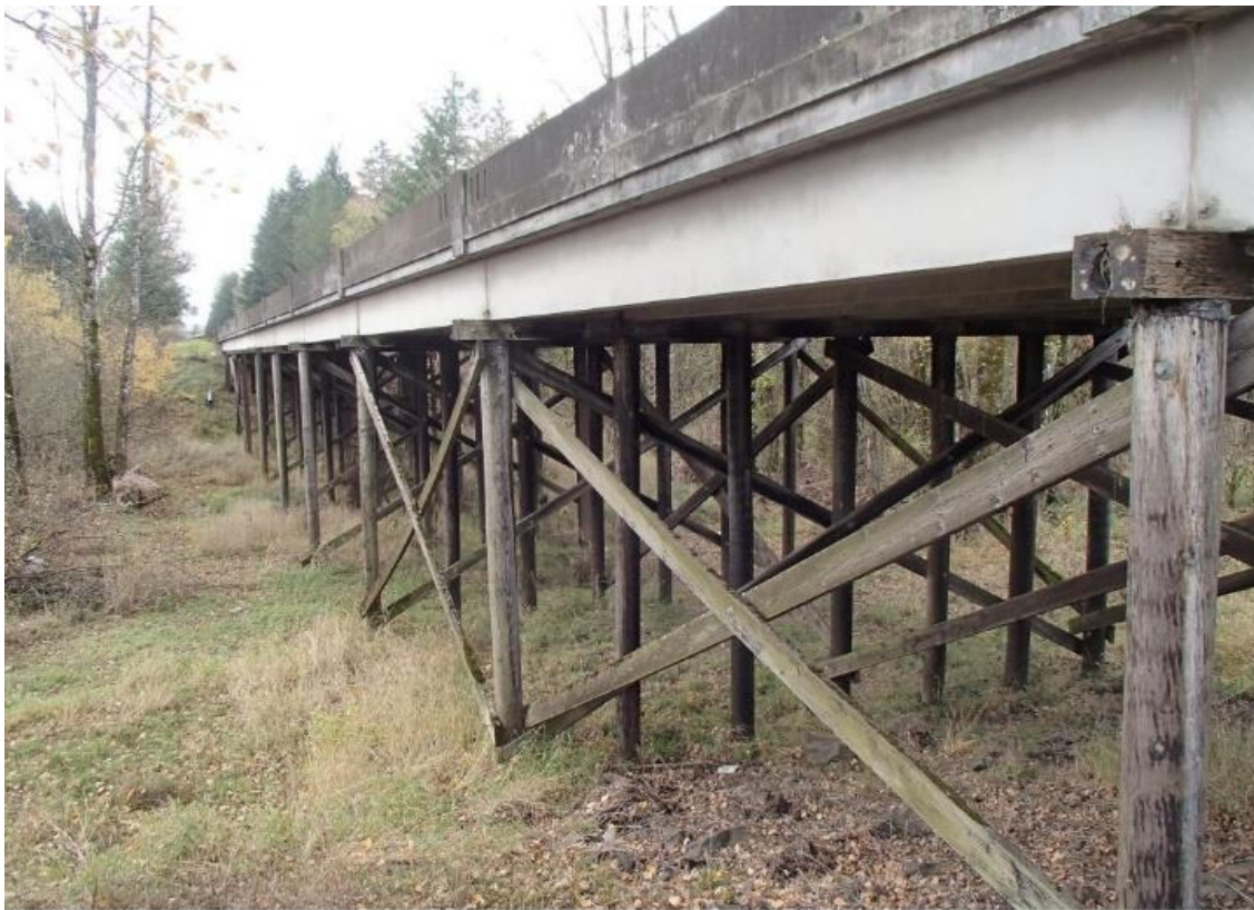
YAMHILL RIVER OVERFLOW - BR# 08492 - HWY 39 - MP: 45.76
