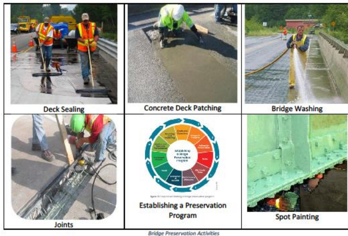
Bridge Preservation Activities
